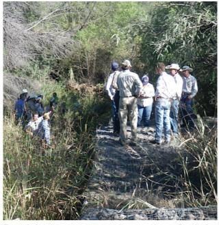
Figure 3. Chihuahua ranchers standing on gabions at Rancho San Bernardino see how this type of erosion control is filling in incised arroyo with sediment and contributing to revegetation of formerly barren channel. Photo: Tom Barry.
