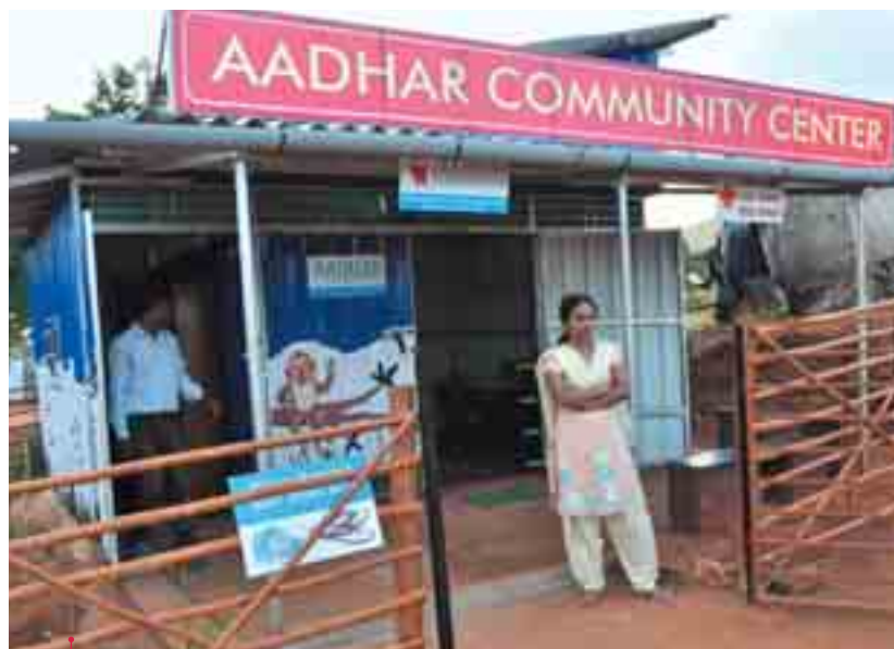
Integrated Energy Centre in Kanbargi with Mahesh Foundation serves as a solar powered community centre with education and health facilities, in addition to being a charging station for lights and mobile phones - Source: SELCO Foundation
