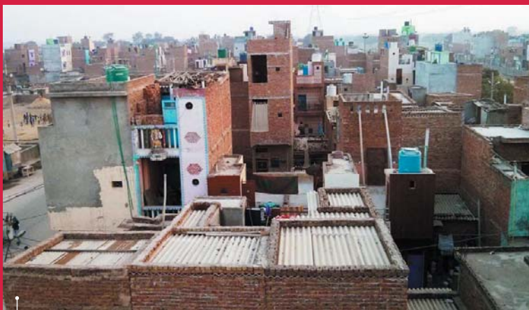
A self-built Informal settlement in Delhi. Source: mHS CITY LAB
