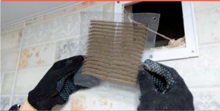
Replacement of a ventilation filter
