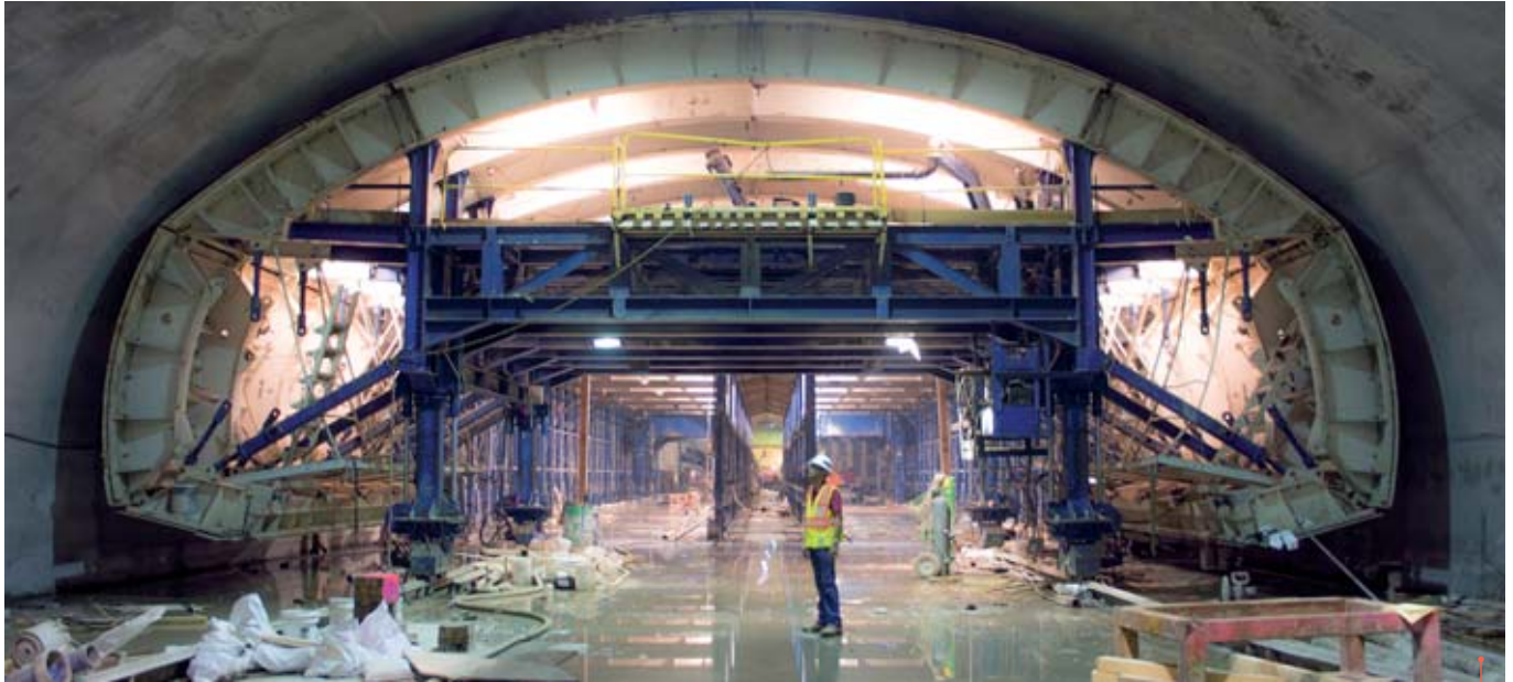
Second Avenue Subway in the making, New York, 2013. MTA Capital Construction/Rehema Trimiew/Wikimedia, © BY-SA
