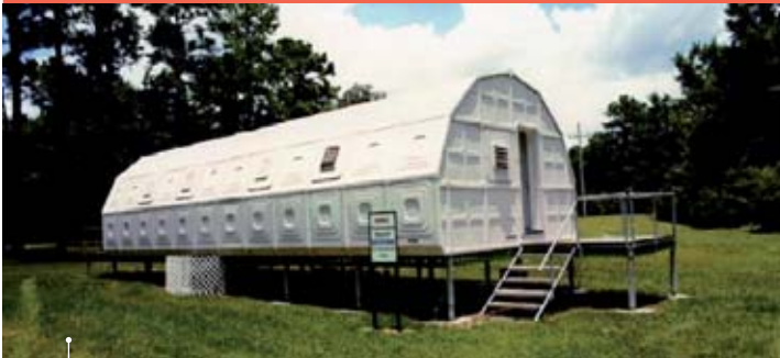
The Biohome, a sealed chamber facility created by NASA in the late 1980s to investigate interior plants' ability to purify the air. © Bill Wolverton
