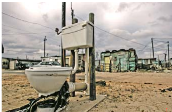
Unenclosed toilet in Cape Town - ©Jaco Marais from online
