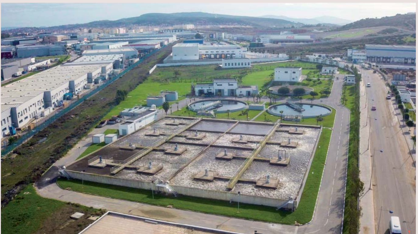
Boukhalef wastewater treatment plant operated by Amendis - ©Veolia
