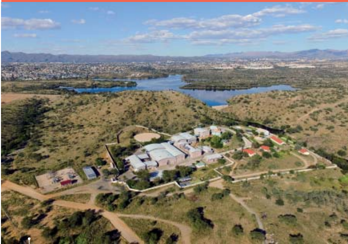
Windhoek wastewater recycling plant - ©Veolia
