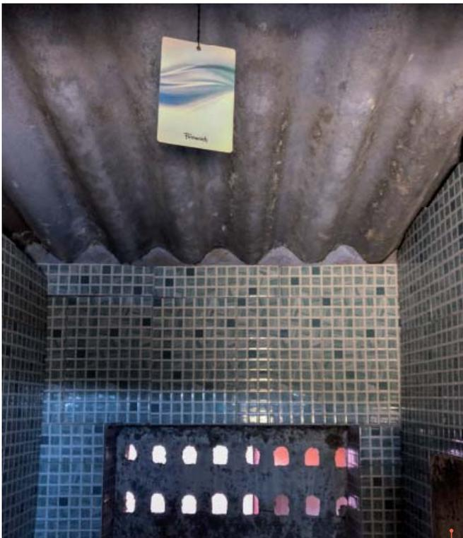
An air-freshener pad treated with the Firmenich-Gates malodor counteractant technology installed in a community toilet for the test. The pad captures malodorous molecules and in turn releases a pleasant fragrance - © Archipel&Co/ Maja Bialon
