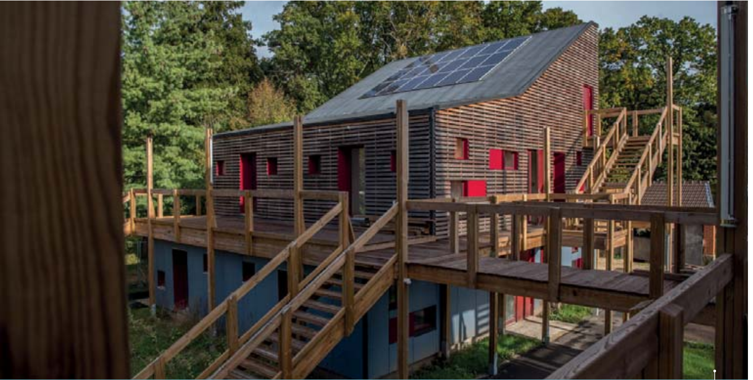
Timber-framed house with solar power, Bouray-sur-Juine, 91 - ©AREC
