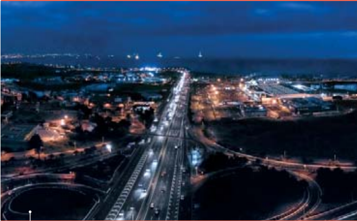
Lighting renovation - ©Signify
