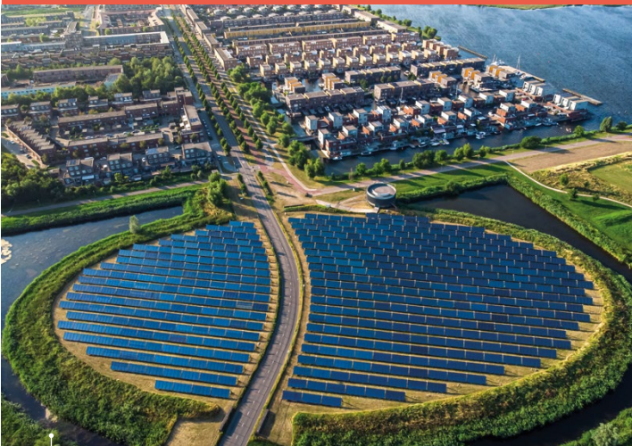
Modern sustainable neighbourhood in Almere, The Netherlands. The city heating (stadswarmte) in the district is partially powered by a solar panel island (Zoneiland). Aerial view.
