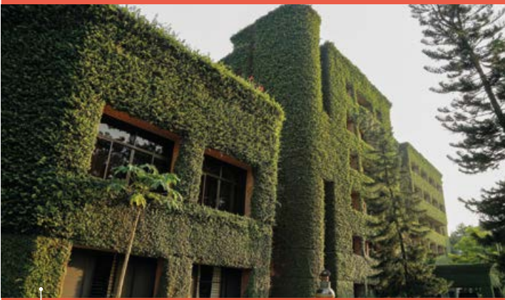
Building of RDRS (Rangpur Dinajpur Rural Service) is covered with green plants in Rangpur - a NGO working to empower the rural poor in northern Bangladesh 02 May 2017. Source: Abir Abdullah / Climate Visuals Countdown.
