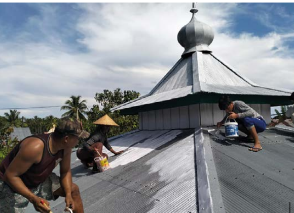
Workers painting a roof with BeCool solar-reflective paint
